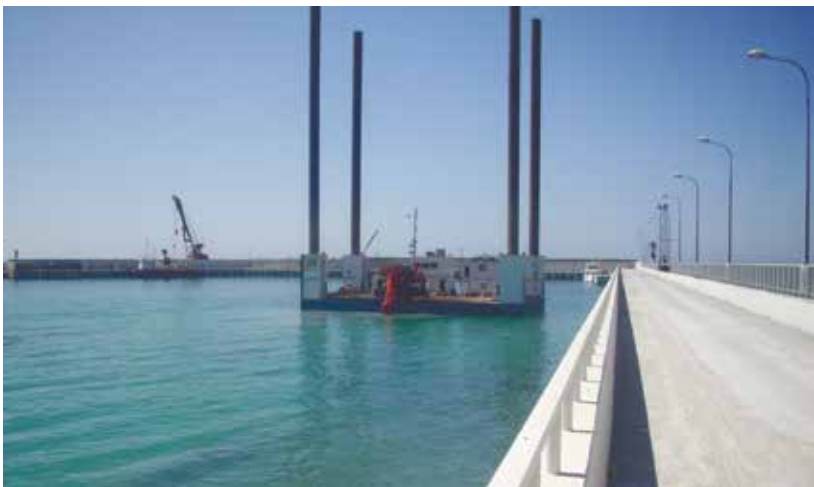
Pile pier construction
